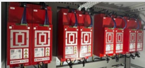
Eight active energy management devices of the PxtRX type generate the necessary power for the short-term UPS.
