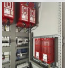
Safe discharge units SDU: For maintenance purposes.
